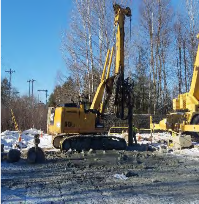
Fig 1: MJ drilling Str. 48. Viewing west. (01-09-20).
