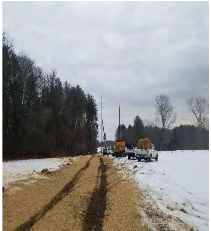
Fig 10: Access road to Str. 105. Viewing east. (01-11-20).
