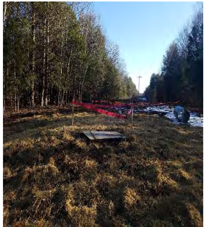
Fig 28: Foundation can set for Str. 73. Viewing east. (01-15-20).
