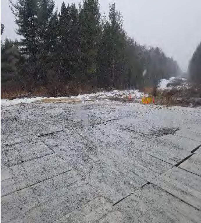
Fig 17: Soil pile removed from Str. 85 work pad. Viewing south. (01-13-20).
