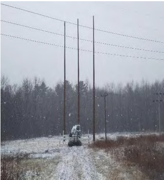
Fig 15: Foundation poles for Str. 143. Viewing west. (01-13-20).
