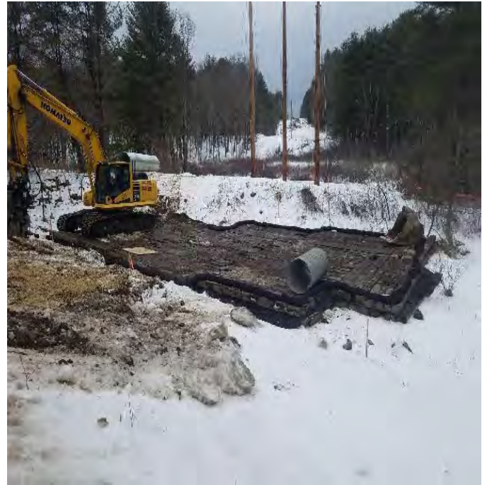
Fig 6: Work pad for Str. 3162-18 in wetland DW100. Viewing east. (01-10-20).
