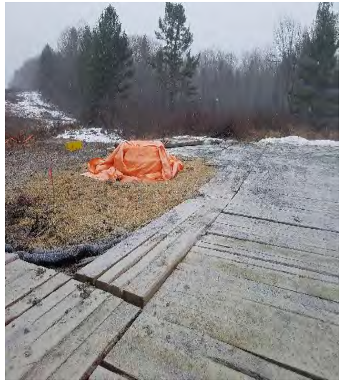
Fig 18: Poured foundation for Str. 85. Viewing south. (01-13-20).
