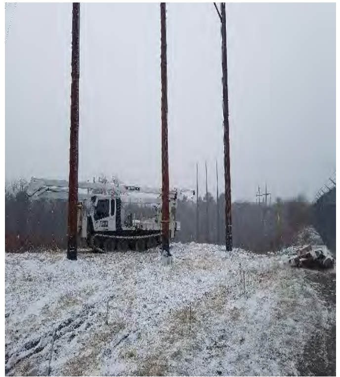
Fig 16: Foundation poles for Str. 144. Viewing west. (01-13-20).
