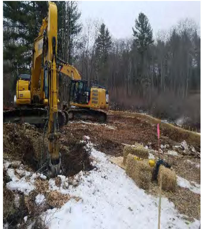
Fig 20: Crew excavating foundations for Str. 60. Viewing east. (01-13-20).
