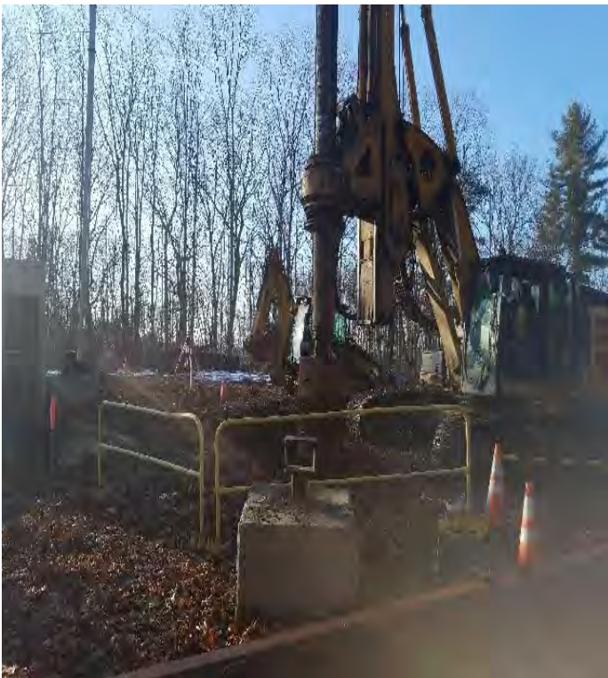
Fig 27: MJ drilling foundations for Str. 58. Viewing southwest. (01-15-20).
