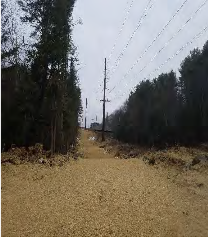
Fig 25: Strs. 10 and 9. Viewing north. (01-14-20).
