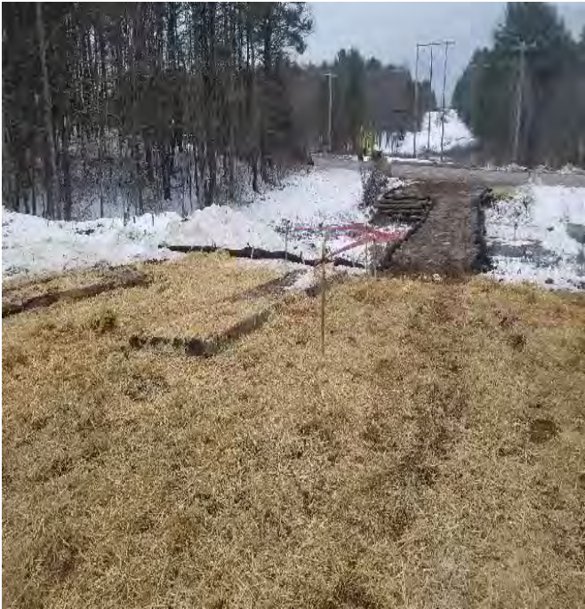
Fig 5: Crew set foundation cans and restored area around Str. 59. Viewing east. (01-10-20).
