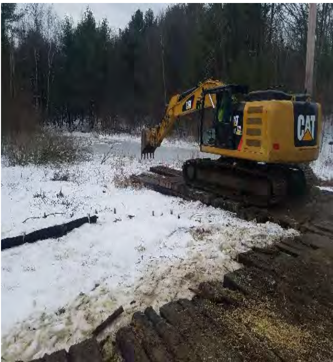
Fig 7: Crew building work pad for Str. 102. Viewing south. (01-11-20).
