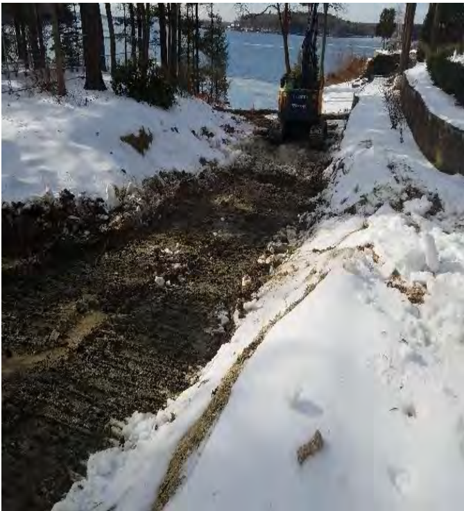
Fig 3: Removing timber mats from Gundalow landing/east side of the Bay. (01-10-20).
