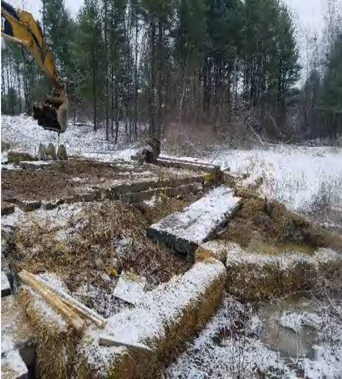
Fig 21: Crew setting foundation can for Str. 102. Viewing south. (01-14-20).
